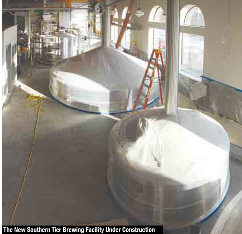
The New Southern Tier Brewing Facility Under Construction
